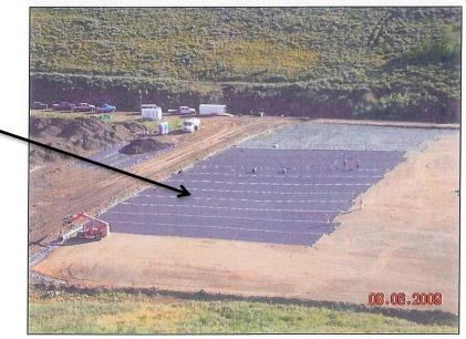
Photo 4. 60-mil HDPE Drainliner™ deployment along north side.
