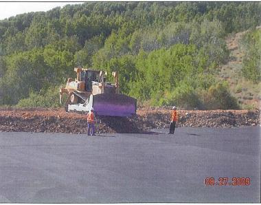
Geocomposite and geofabric placed along road and east drainage
