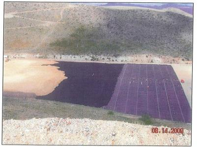
Photo 6. HDPE liner, geofabric and cover fill placement on regraded heap, looking east.
