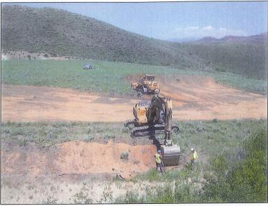
Photo 1. Exposing existing liner edge and dozer stripping topsoil.
