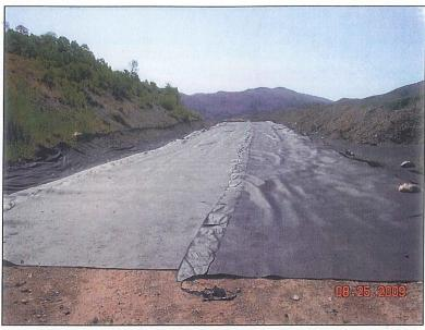
Photo 7. Geocomposite and geofabric placed along road and east drainage, looking south.
